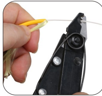
3. Remove 0.9mm cable jacket 50mm.
